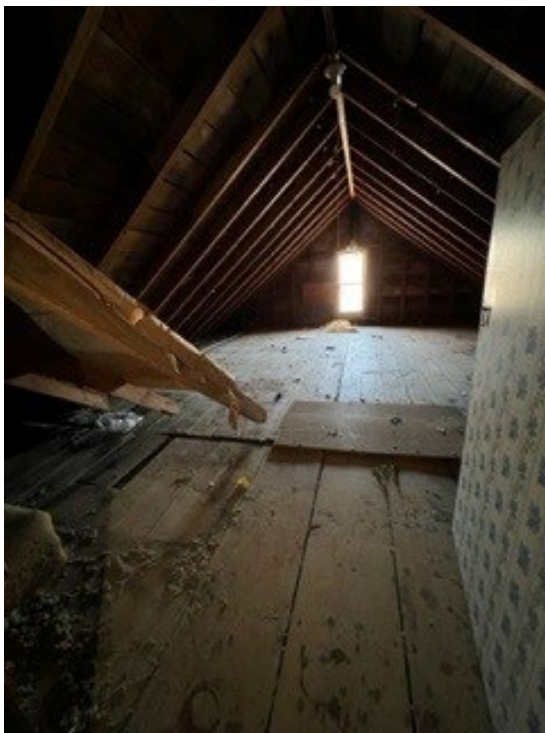
Unfinished Attic Space
