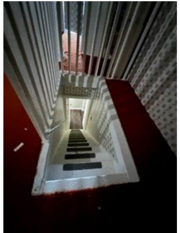
Stairs to Attic
