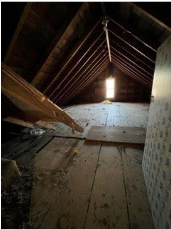
Unfinished Attic Space
