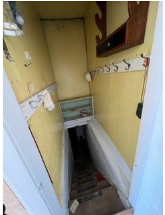
Stairs to Basement
